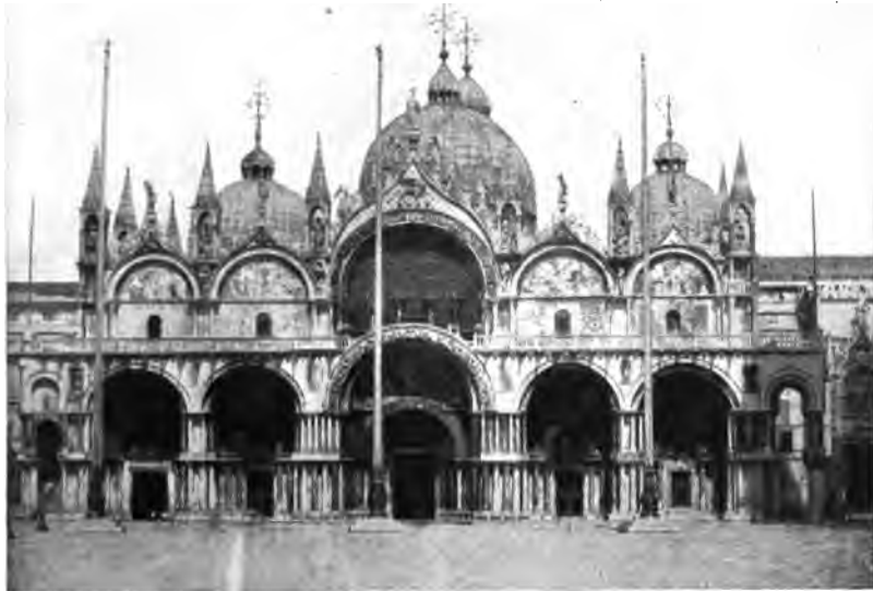
THE MOST IMPORTANT MONUMENT OF BYZANTINE ARCHITECTURE The use of arches and short columns is essentially Byzantine, as also the rich decorations in fresco and mosaic (The Cathedral of St. Mark, Venice)
